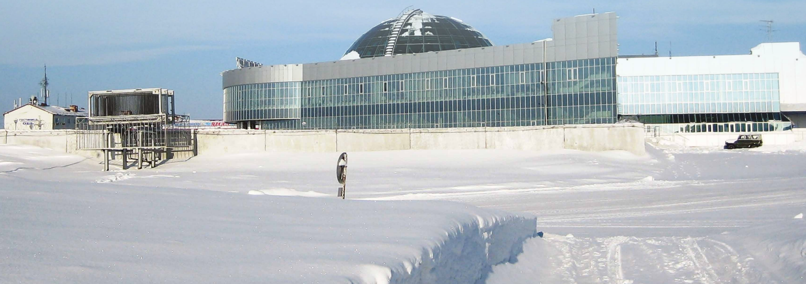
Salekhard Airport with the VET temperature stabilization system at the base of the terminal building
